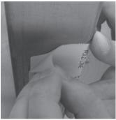
3. Carefully cut the frame inside the un-shaded area marked on the template. Install strike per installation instructions A89071.
