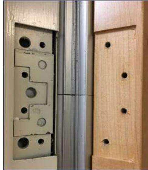
**NOTE! Covers of the upper part of the hinge are slightly shorter than the hinge. When installing bottom hinge covers push the covers up to eliminate any gap.**
