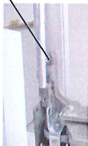
Top latch fully extended and deadlatched. Rod shown is too long. Adjust upward by rotating counter clockwise until flush with bell crank.
