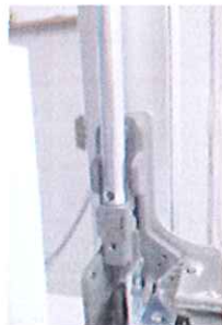
Top latch fully extended and deadlatched. Rod fully extended and flush with bell crank.
